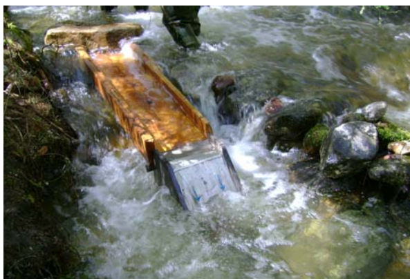
Intake box with hydro screen
