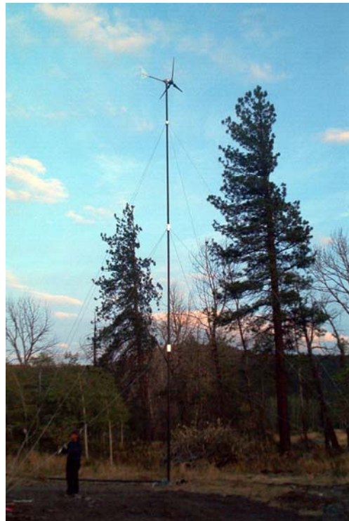
Wind Turbine in Merritt, BC
